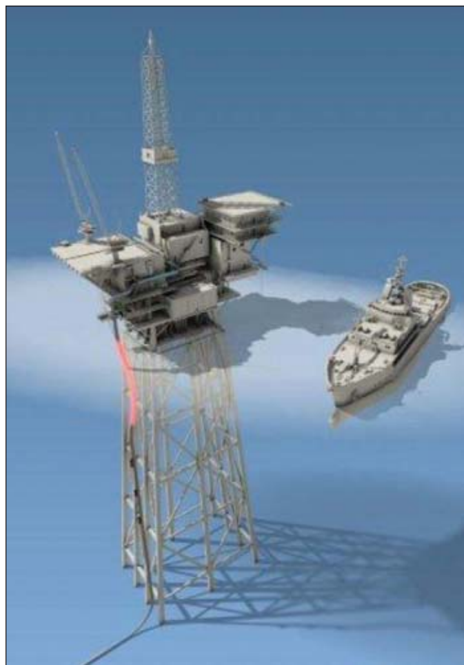
In 2007 a vessel collided with the southeast face of satellite platform jacket, damaging the 12-in. OD export riser (highlighted in red). The impact damaged the riser and a large portion of the connected topside pipeworks (Fig. 1).
